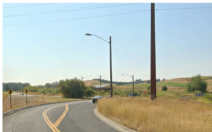
Airport Road at Terre View Road.
